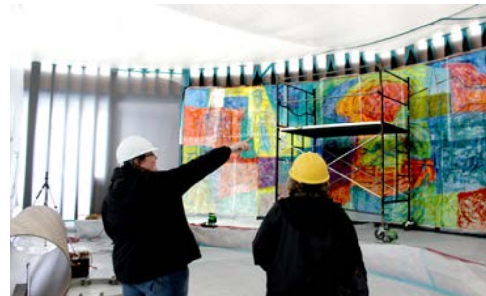
LRAPA employees visit the Eugene City Hall asbestos abatement site.
