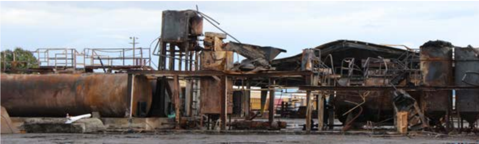
Swanson Mill during asbestos abatement after the July 2014 fire.
