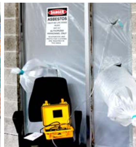
Proper asbestos abatement equipment.
