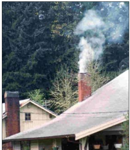
A smoky chimney indicates improper use of a wood stove/fireplace and emits excess pollution into the air.
