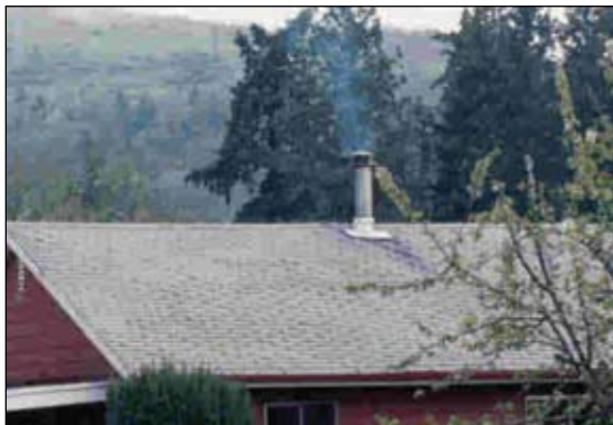
Chimney smoke should be negligible when a wood stove/fireplace is being properly used.
