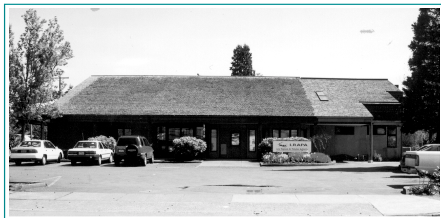
LRAPA's newly remodeled administrative office at 1010 Main Street in Springfield. The laboratory addition on the right side of the building was completed in Fall '99.
